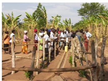
Opening a borehole
